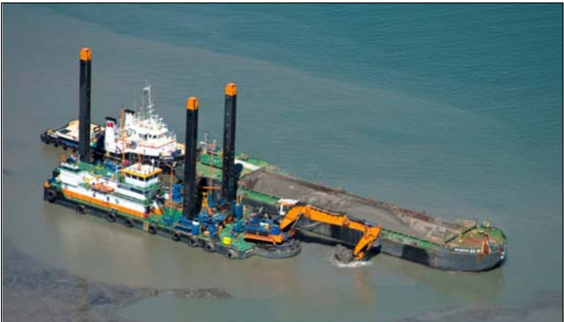
Plate 2.2 Example of a BHD, filling a dumb barge with assisting tug, (photograph courtesy of GLNG)
