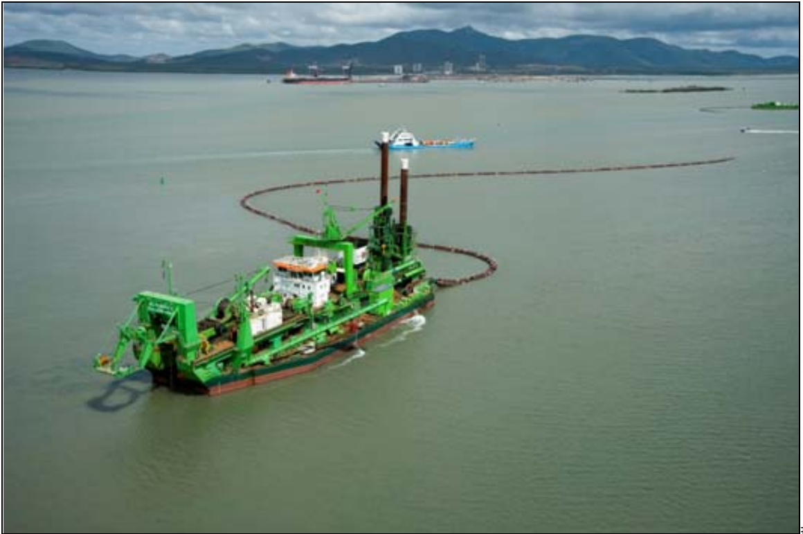
Plate 2.3 Cutter Suction Dredger with floating pipeline connect, (photograph courtesy of GLNG)
